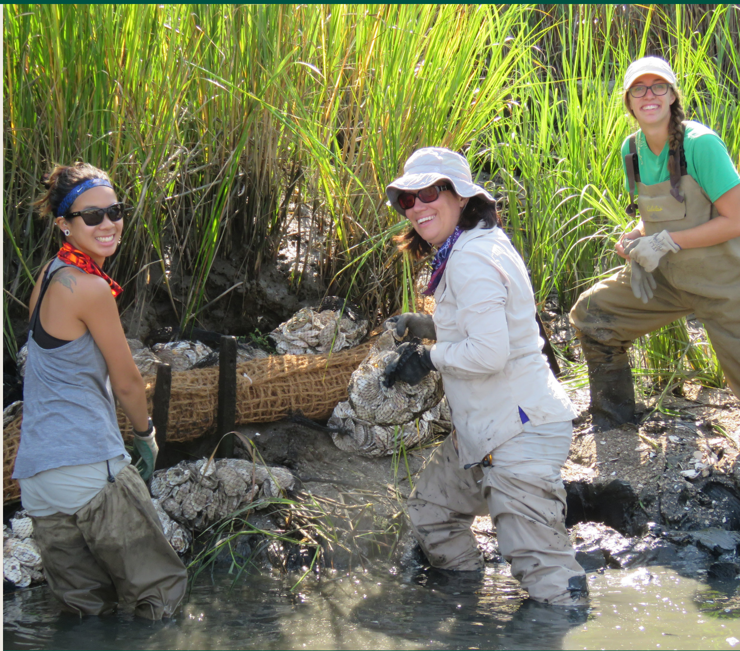
Installation of a living shoreline along the Nantuxant Creek in NJ. | Credit: PDE
